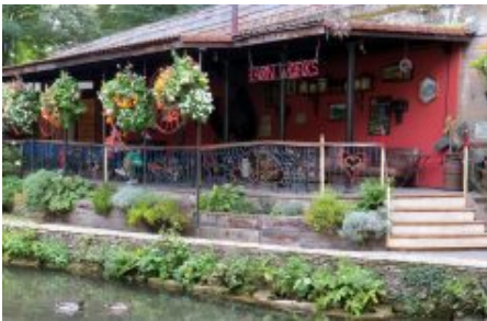
Egypt Mill Terrace
